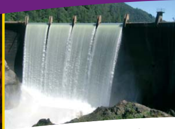
Dam wall monitoring
